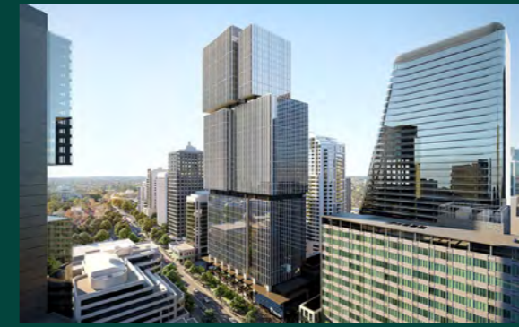
Victoria Cross Over Station Development, Sydney Australia
